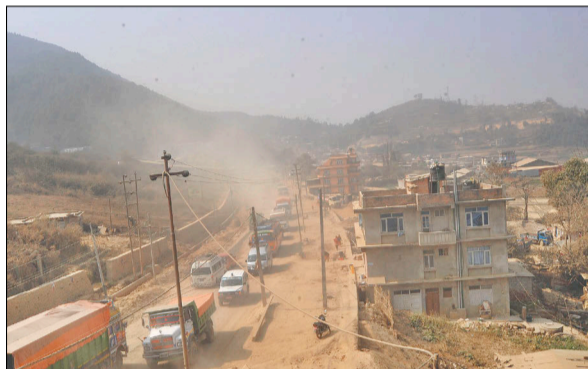
■ A dusty section of the Kalanki-Satungal road. POST FILE PHOTO
