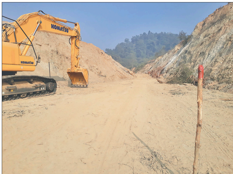
Construction works at a section of the Kathmandu-Tarai Expressway.
