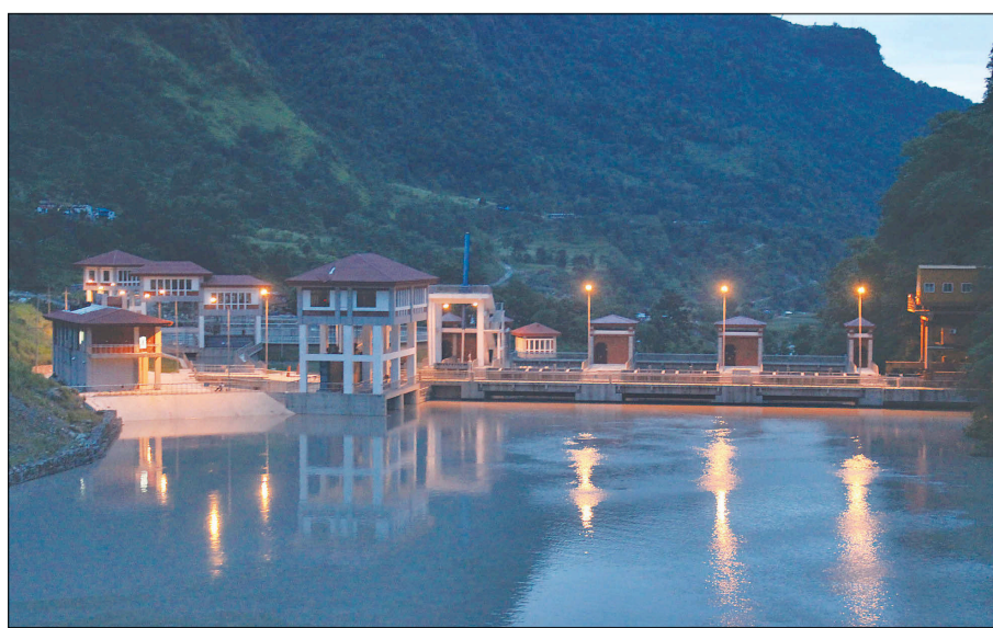
A general view of Upper Marsyangdi A Hydropower Plant in Lamjung.
