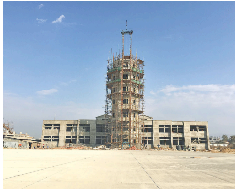
A general view of the under construction control tower in Bhairahawa.
