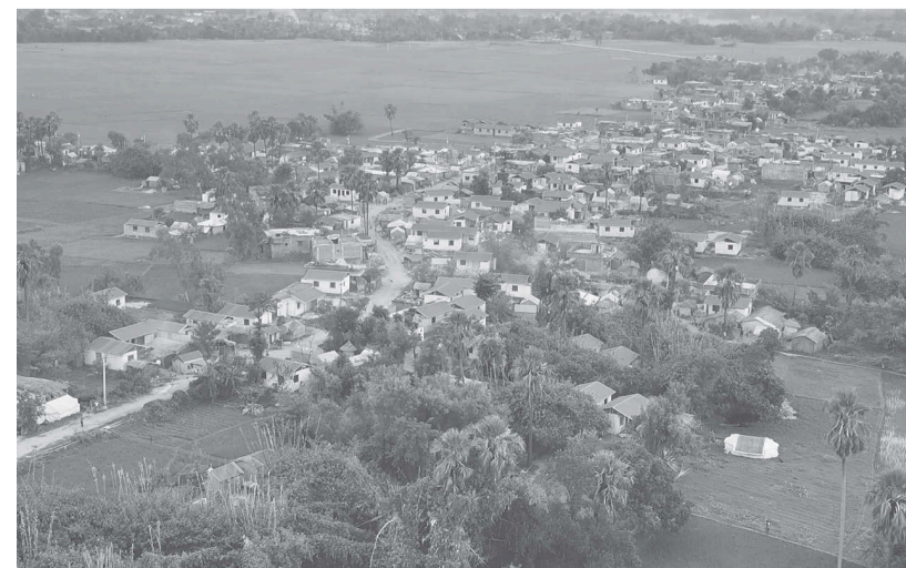
The homes were built by the Nepal Army for the families displaced by the windstorm.
