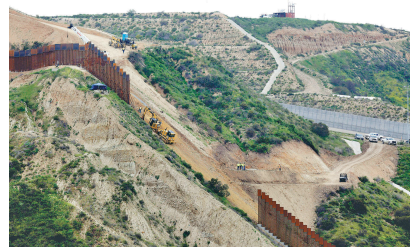
In this March 11, 2019 photo, construction crews replace a section of the primary wall separating San Diego, above right, and Tijuana, Mexico, below left, seen from Tijuana, Mexico. AP/RSS
