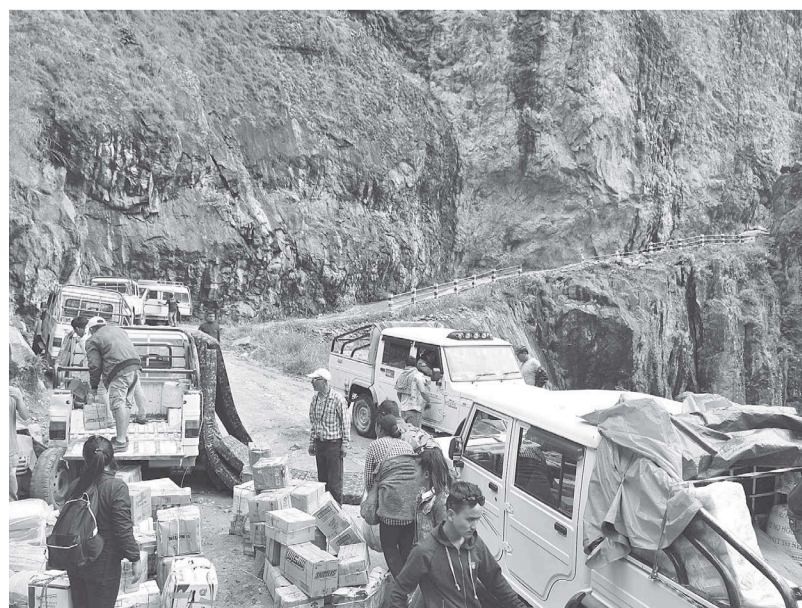
The Besishar-Chame road sees frequent landslides due to the region's weak topography.
