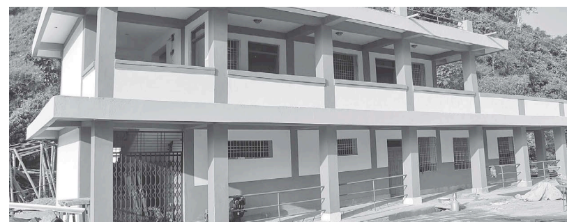
The 15-bed hospital in Sanibheri Municipality has completed construction.
