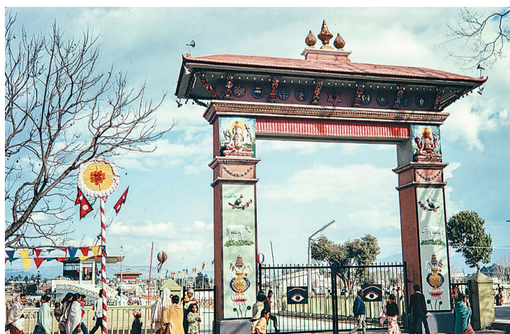
A gate under construction at Tundikhel for the coronation of King Birendra.
