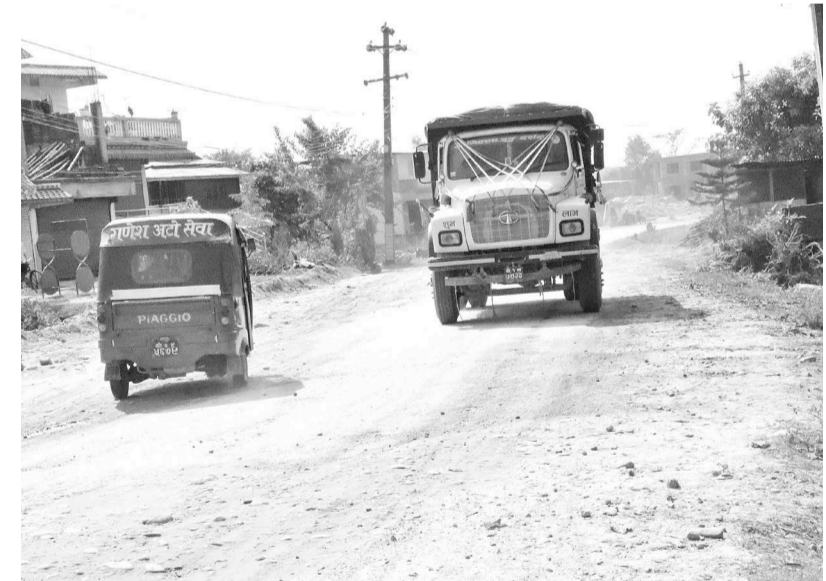
As a short-term solution, locals have resorted to sprinkling water on the road and the nearby areas.
