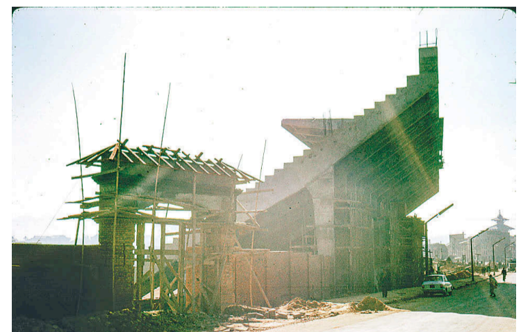
The National Stadium under construction in 1975.
