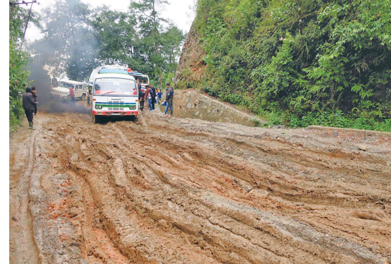
Road upgradation work along Lamosanghu-Jiri has remained incomplete for four years.
