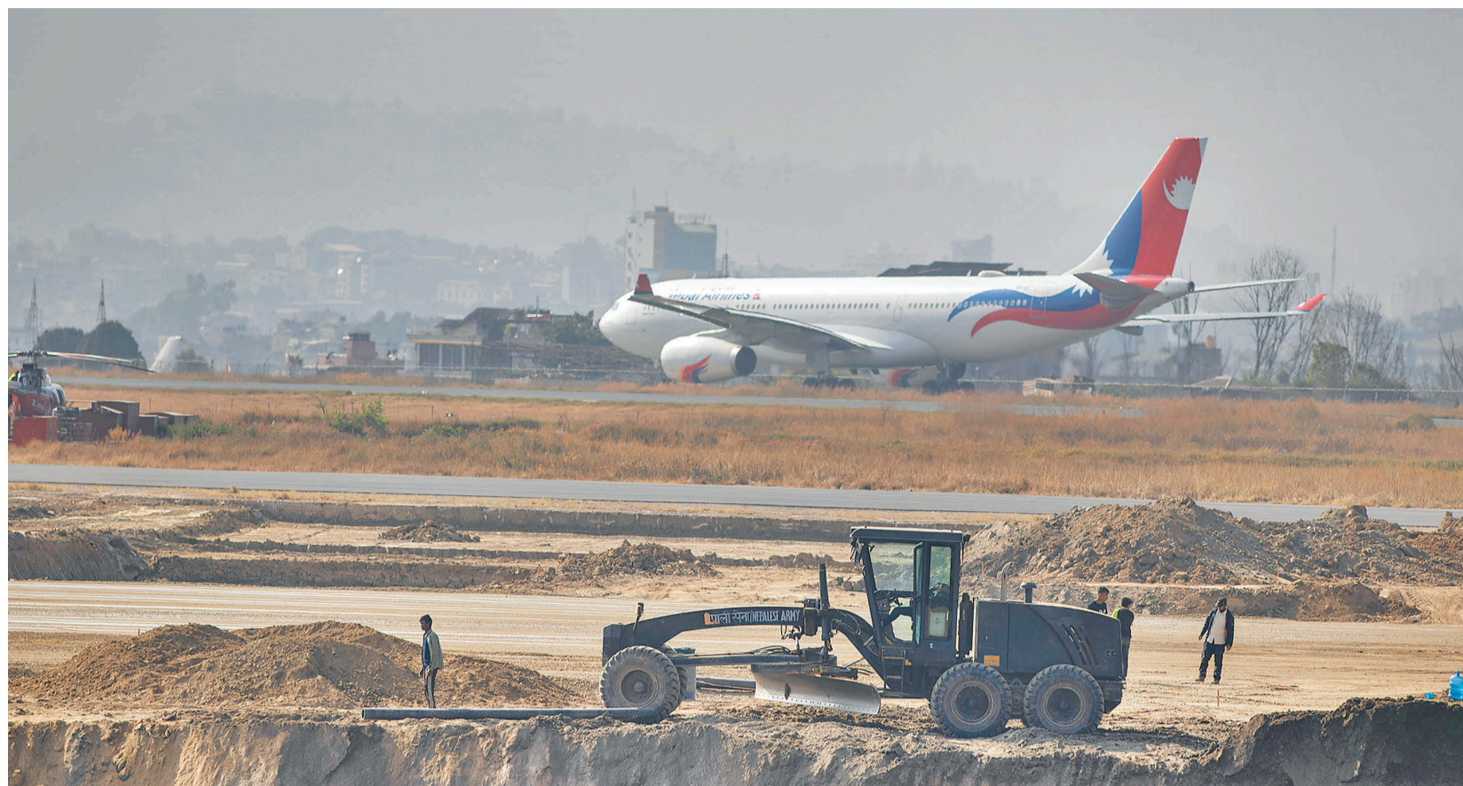
A view of a construction site at Tribhuvan International Airport.
