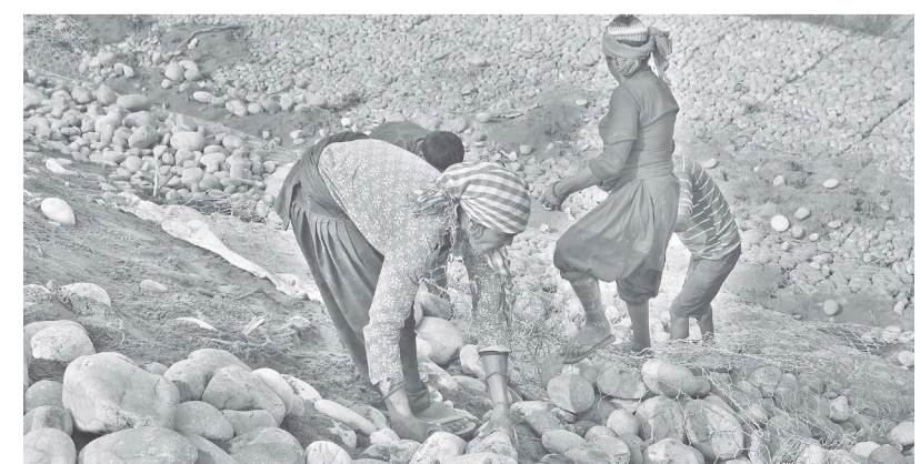
Workers are making up to Rs 1,200 per day filling nets with stones on the river bank.
