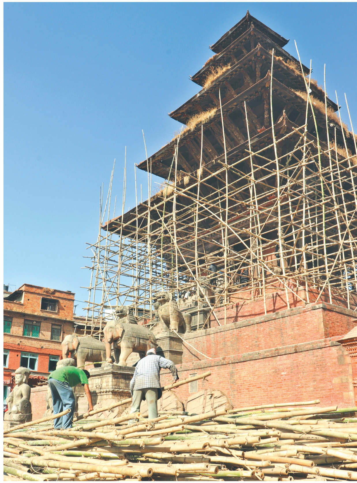
Workers build a bamboo scaffold to clean Nyatapola Temple in Bhaktapur.
