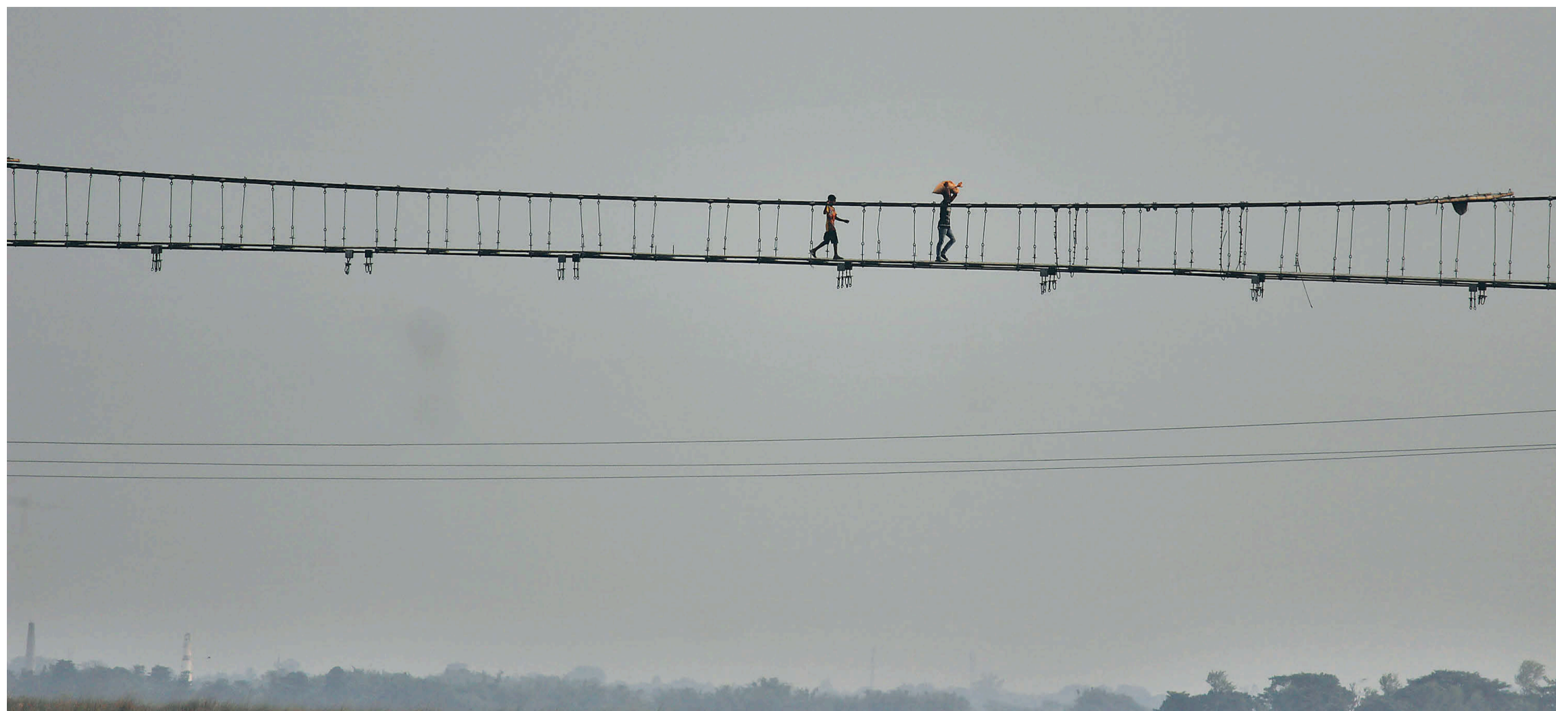
Two figures seen crossing a suspension bridge in Bhadrapur, Jhapa.
