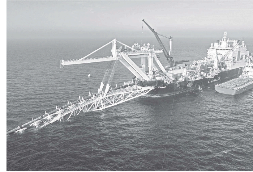
An aerial view of the ship 'Audacia', from where parts of the Nord Stream 2 pipeline are laid in the Baltic Sea off the coast of the island of Ruegen, northeastern Germany.
