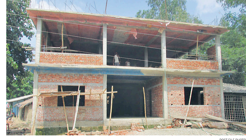
An under-construction municipal office building in Sarlahi district.
