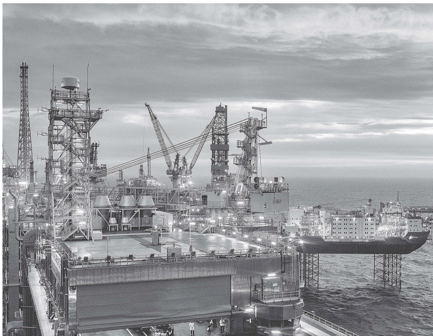
The field centre of the Johan Sverdrup oil field in the North Sea west of Stavanger, Norway, is pictured on Tuesday. Johan Sverdrup, situated some 140 km off the south western coast of Norway and operated by Equinor, is the third largest oil field on the Norwegian continental shelf, with expected resources of 2.7 billion barrels of oil equivalent.
