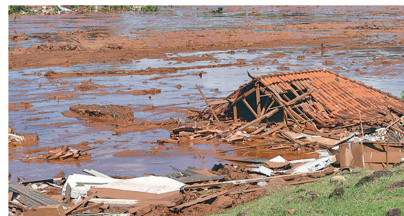
In this January 25, 2019 photo, a structure lies in ruins after a dam collapsed near Brumadinho, Brazil.
