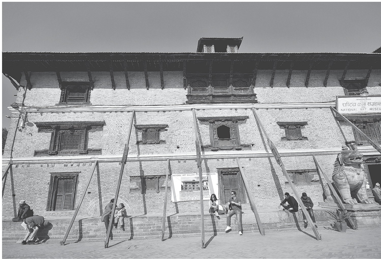
Visitors soak the sun in Bhaktapur Durbar Square on Tuesday.
