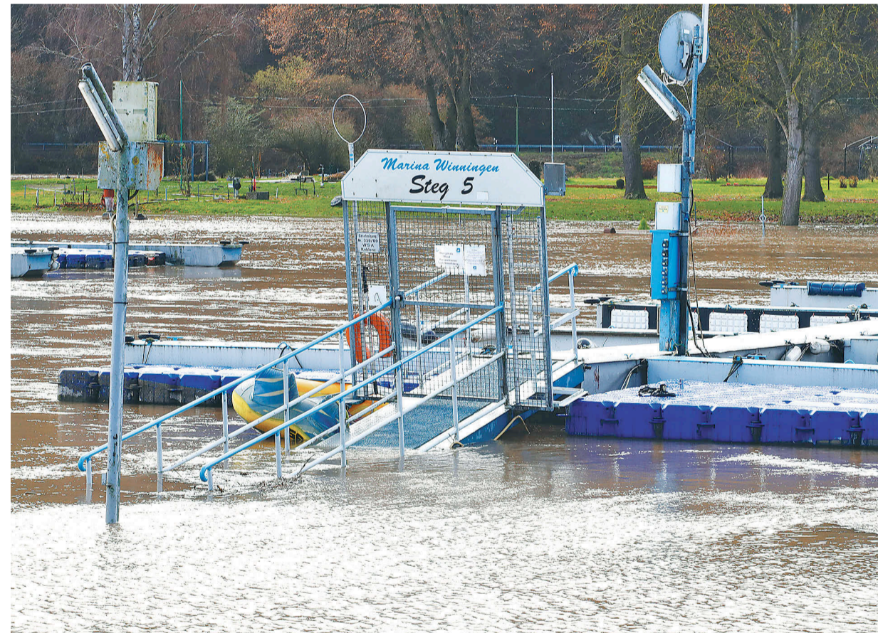
A shipping pier of a sport yachts harbour is flooded by the river Moselle due to heavy rainfalls in western Europe in Winnig near Koblenz, Germany, on Tuesday.
