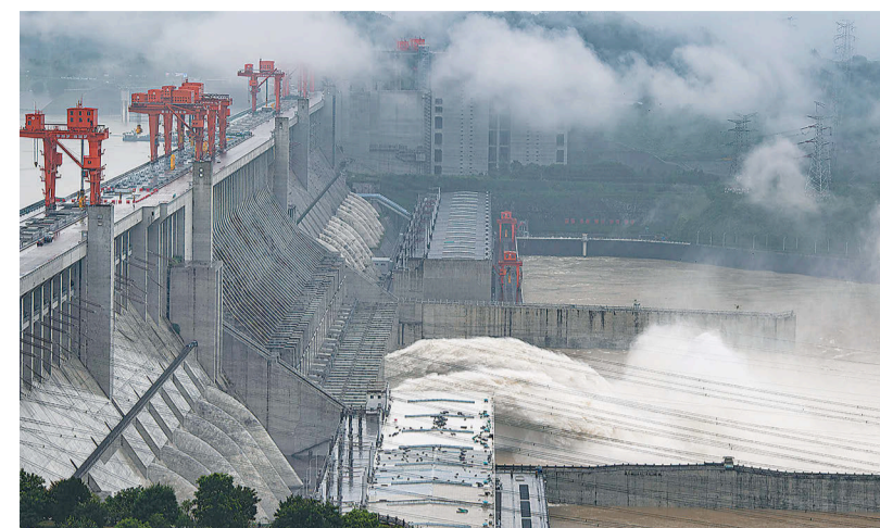
In this photo released by China's Xinhua news agency, water flows out from sluiceways at the Three Gorges Dam on Yangtze River near Yichang in central China's Hubei Province, on Friday.
