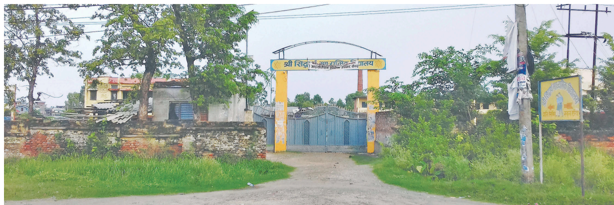
An isolation ward set up at a school building in Birgunj about a month ago has not come into operation as it still lacks proper infrastructure.
