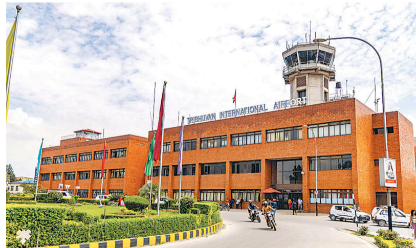
Besides English language skills, the Department of Immigration has also proposed that anyone going abroad on a visit visa must buy insurance worth Rs2 million.
