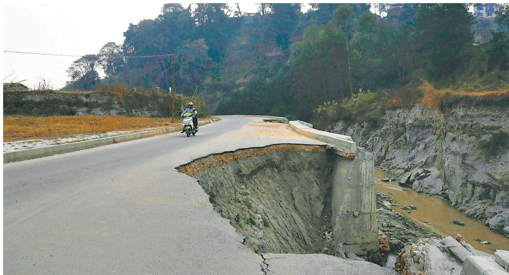
A man rides a scooter near a collapsed road section at Tarkeshwor Municipality, Kathmandu. The section was built just a year ago.
