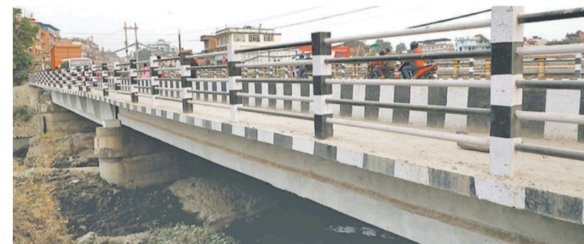
A bridge over Bishnumati river in Teku, Kathmandu built by Pappu Construction. POST FILE PHOTO
