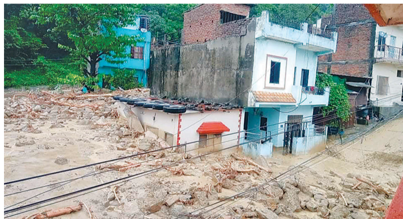
Seven houses were buried in a landslide at Jyotinagar Bamghat in Butwal on Monday.
