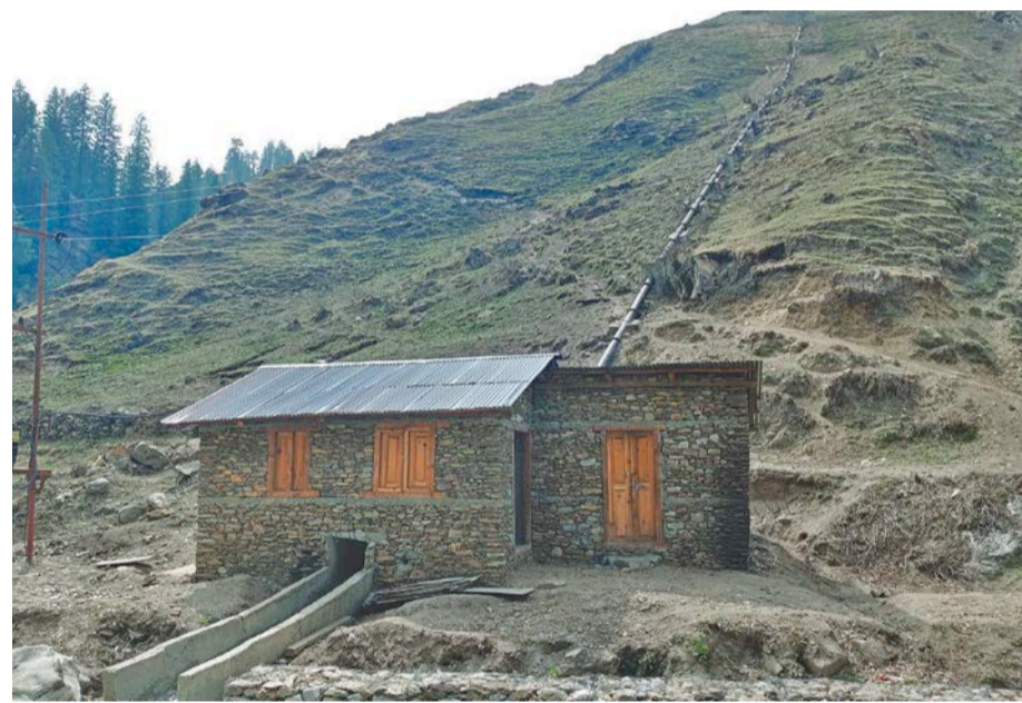
The 42kW Adalikhola Hydropower Project started generation around four months ago.
