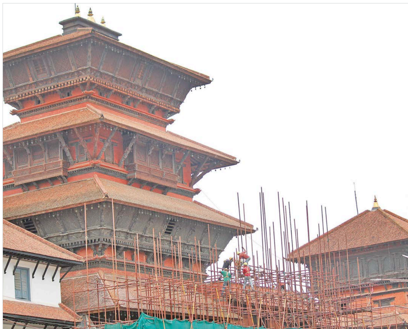
People work on scaffolds at the Nautale Temple, which is undergoing reconstruction, in Basantapur Durbar Square, Kathmandu, on Wednesday.
