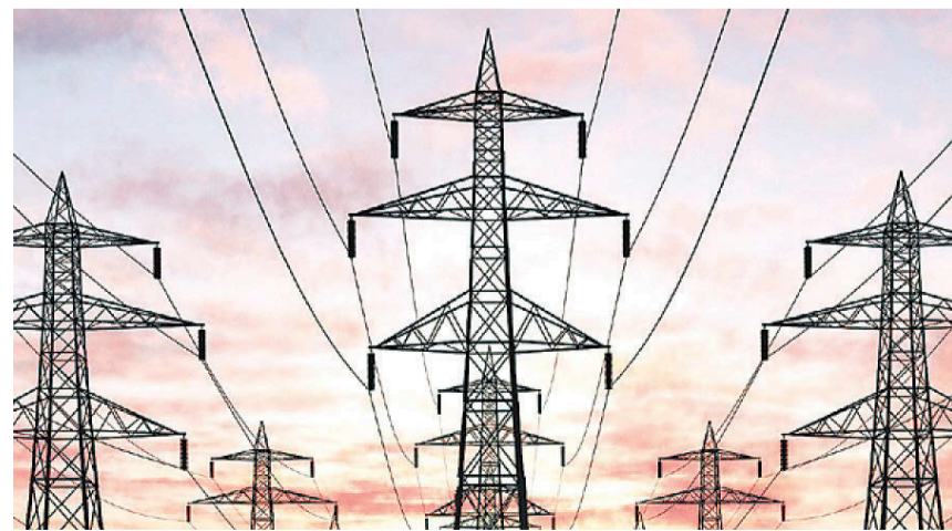
Landslides caused by incessant rainfall have disrupted supply of electricity to factories.
