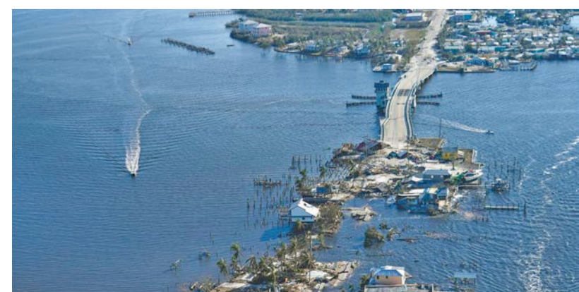
A file photo shows the bridge leading from Fort Myers to Pine Island, Florida heavily damaged in the aftermath of Hurricane Ian.
