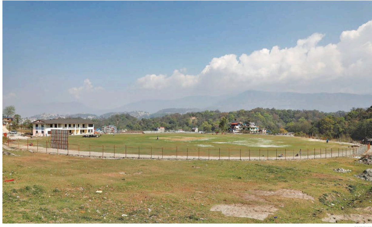
The construction of Mulpani Stadium began as early as 2006, but remains incomplete.
