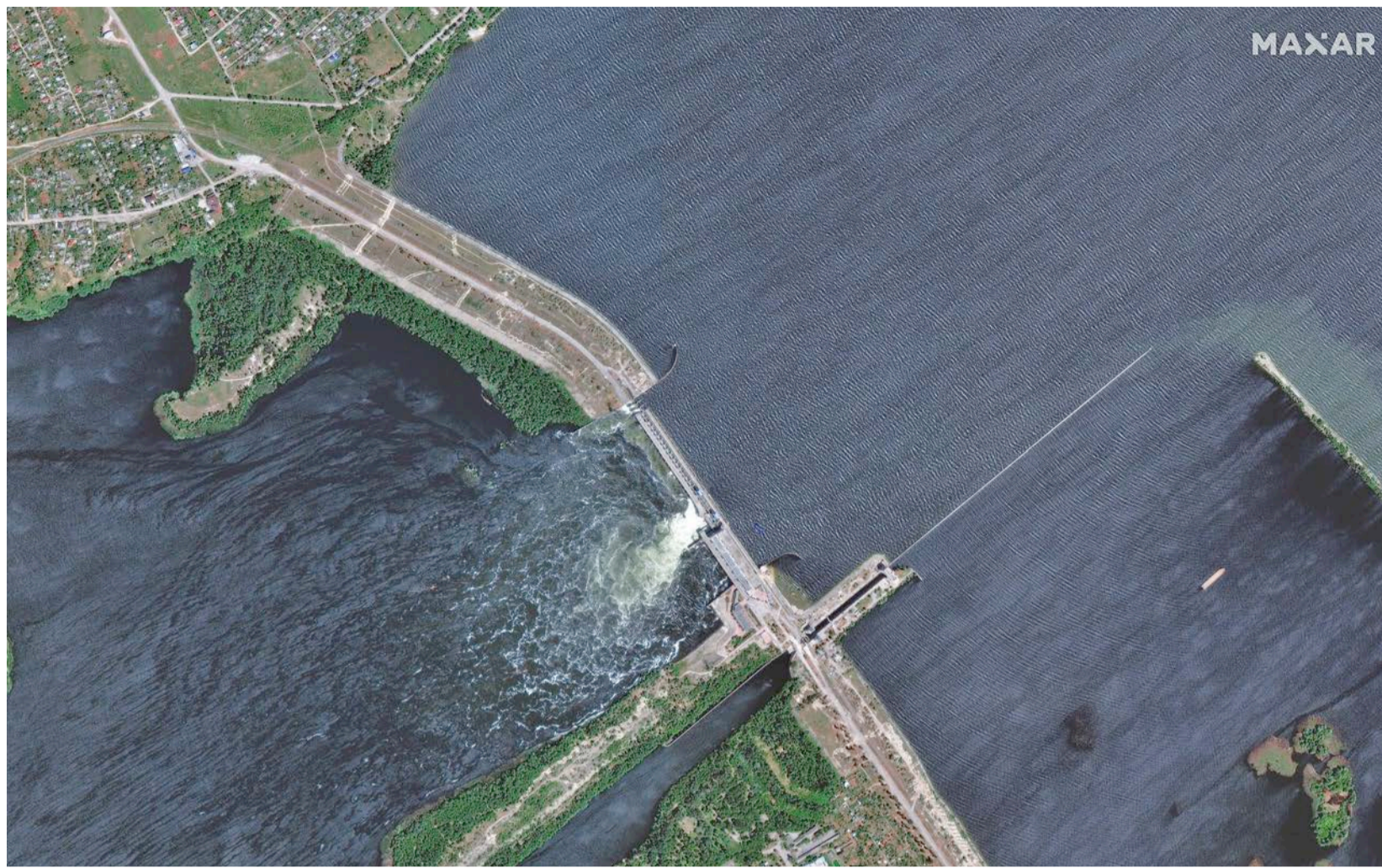
This satellite image provided by Maxar Technologies shows an overview of the Kakhovka dam in southern Ukraine on Monday. Ukraine on Tuesday accused Russian forces of blowing up the major dam and hydroelectric power station in a part of southern Ukraine they control, threatening a massive flood that could displace hundreds of thousands of people.
