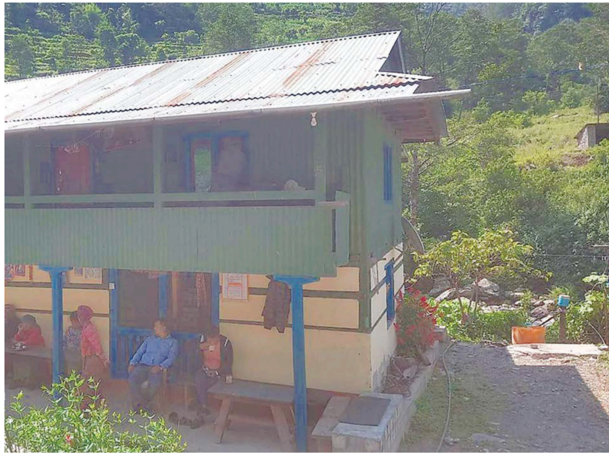
Forty-two families in ward 1 of Pakernas of Umakunda Rural Municipality are reportedly in high risk after a suspected leak in the Likhu-2 tunnel.
