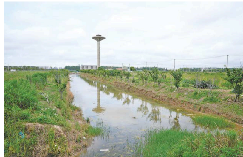
A view of a plot of land designated to be used by Tesla for an expansion of its Gigafactory in Shanghai, China on Monday.
