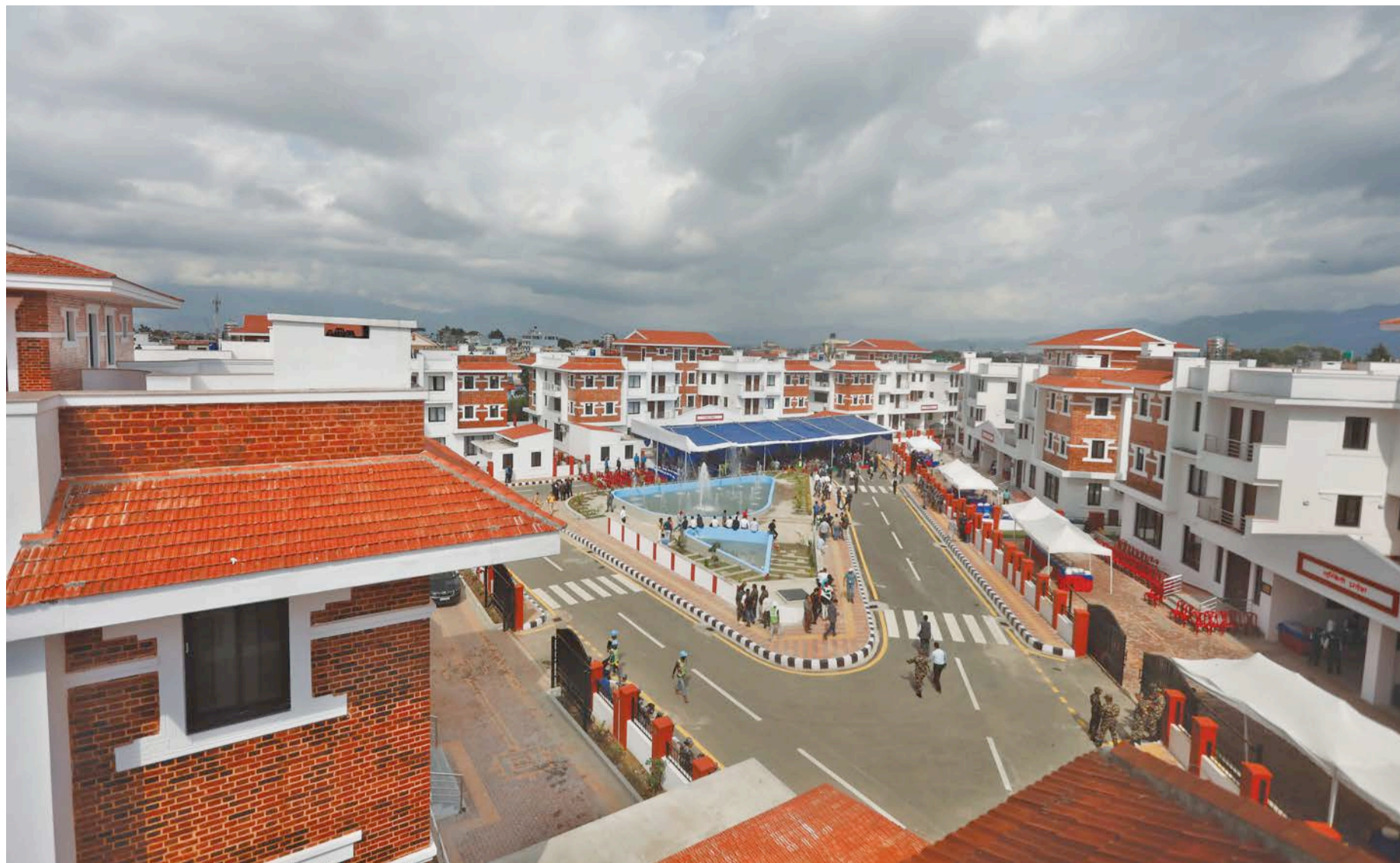
A view of the residences at Bhainsepati in Lalitpur that Prime Minister Pushpa Kamal Dahal handed over to the province heads and chief ministers on Sunday.
