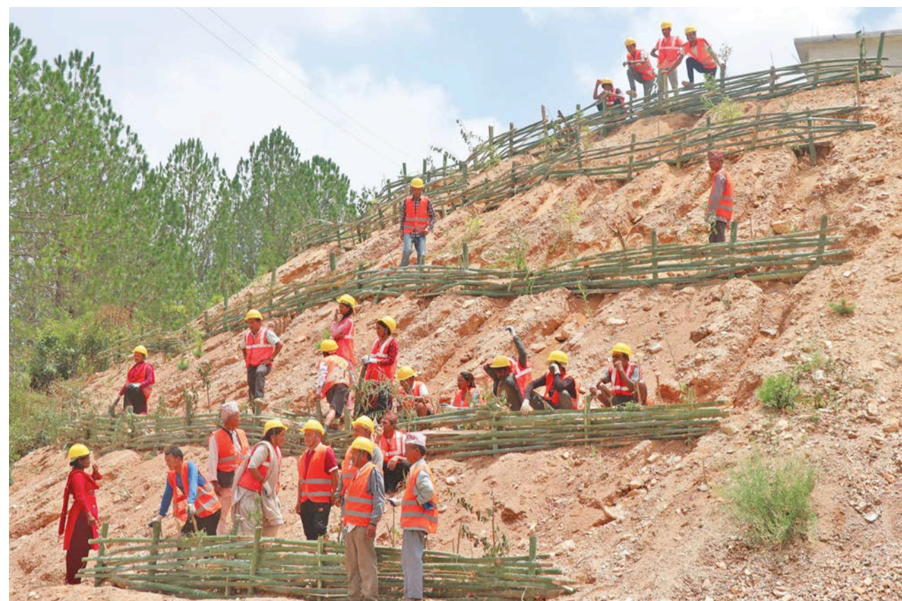
(Left) Workers instal bamboo barriers on a slope to prevent land erosion in Chhatreshwari Rural Municipality in Salyan in this recent photo. (Right) Last year's massive landslide in the middle of a village in ward 5 of Kapurkot Rural Municipality in Salyan district in this recent photo.
