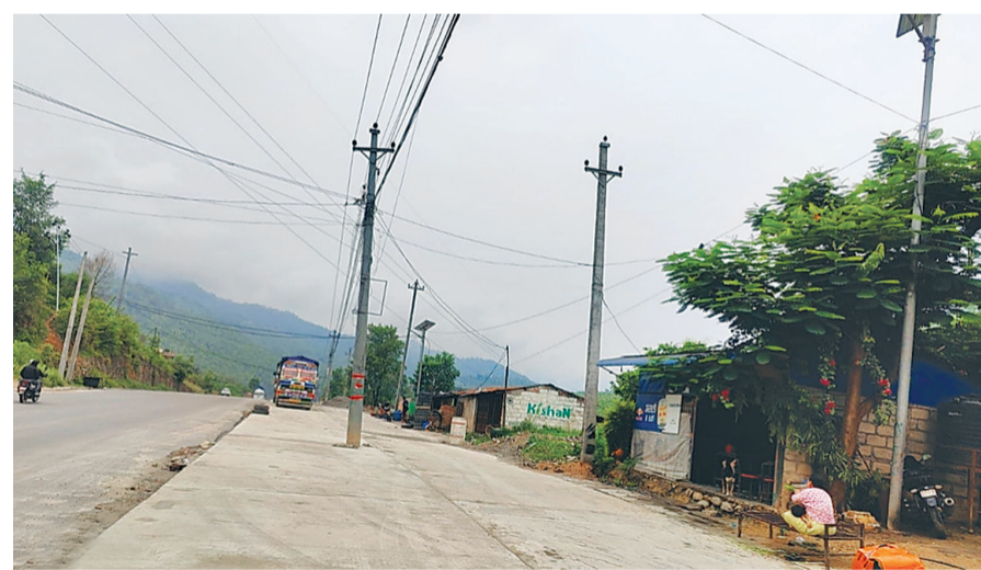
POST FILE PHOTO This undated photo shows an electricity pole standing in the middle of a widened road in a hill district.
